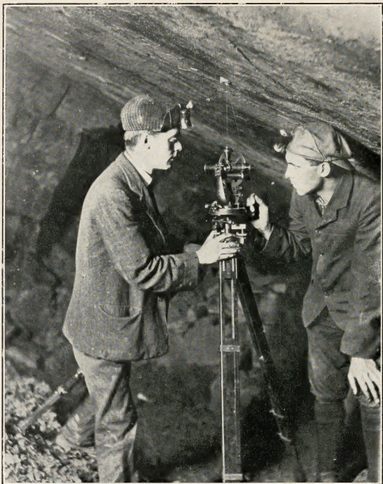
CENTRING A THEODOLITE UNDER A ROOF-STATION IN A MINE.
